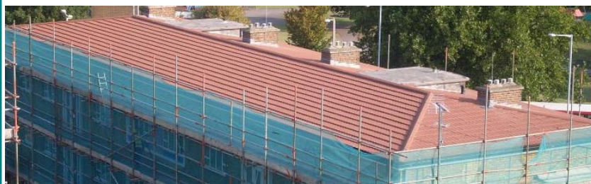
Roof at High Cross and Hale
